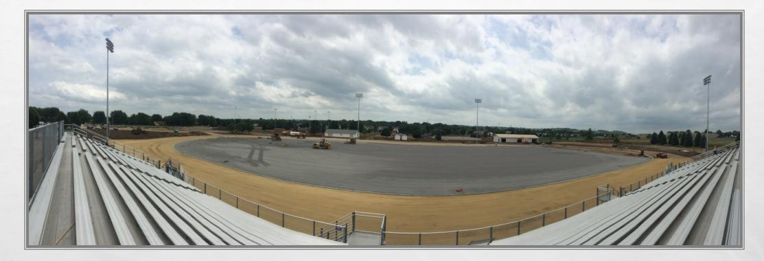
PANORAMIC VIEW OF THE FIELD – ROCK FOR ARTIFICIAL TURF IS BEING INSTALLED, CURBING AROUND FIELD/TRACK AND CLASS 5 AT THE TRACK ARE BEING INSTALLED
