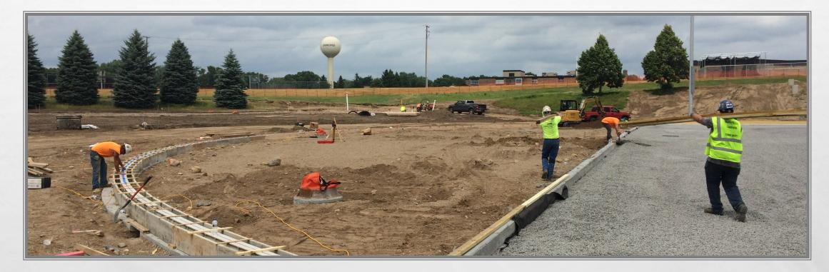
INSTALLATION OF CURB, GUTTER, AND NAILER AT WEST END OF THE FIELD
